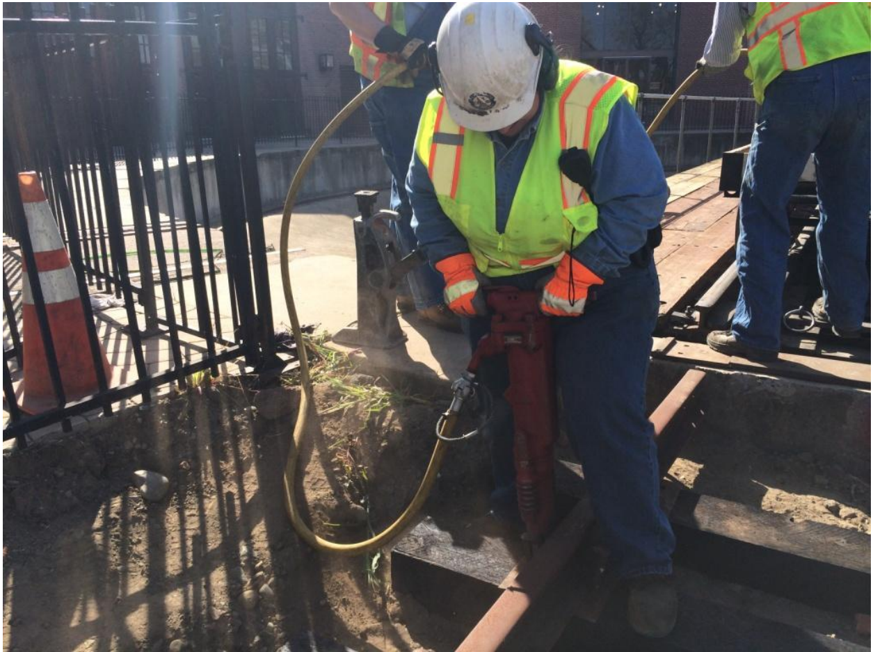
Heather drives the first spike of the new Whisker Track!
