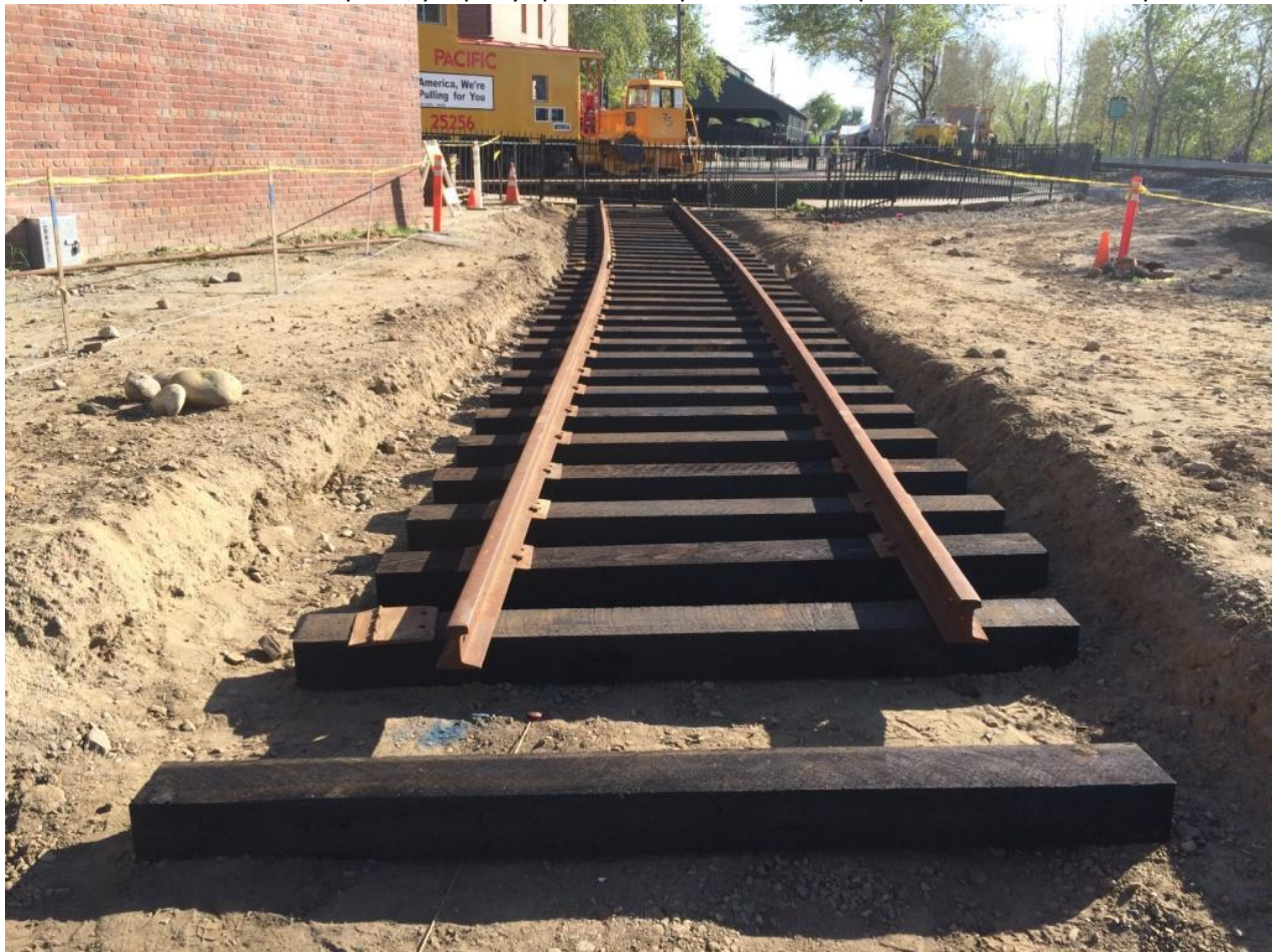
At day's end, it's starting to look like a real railroad track
