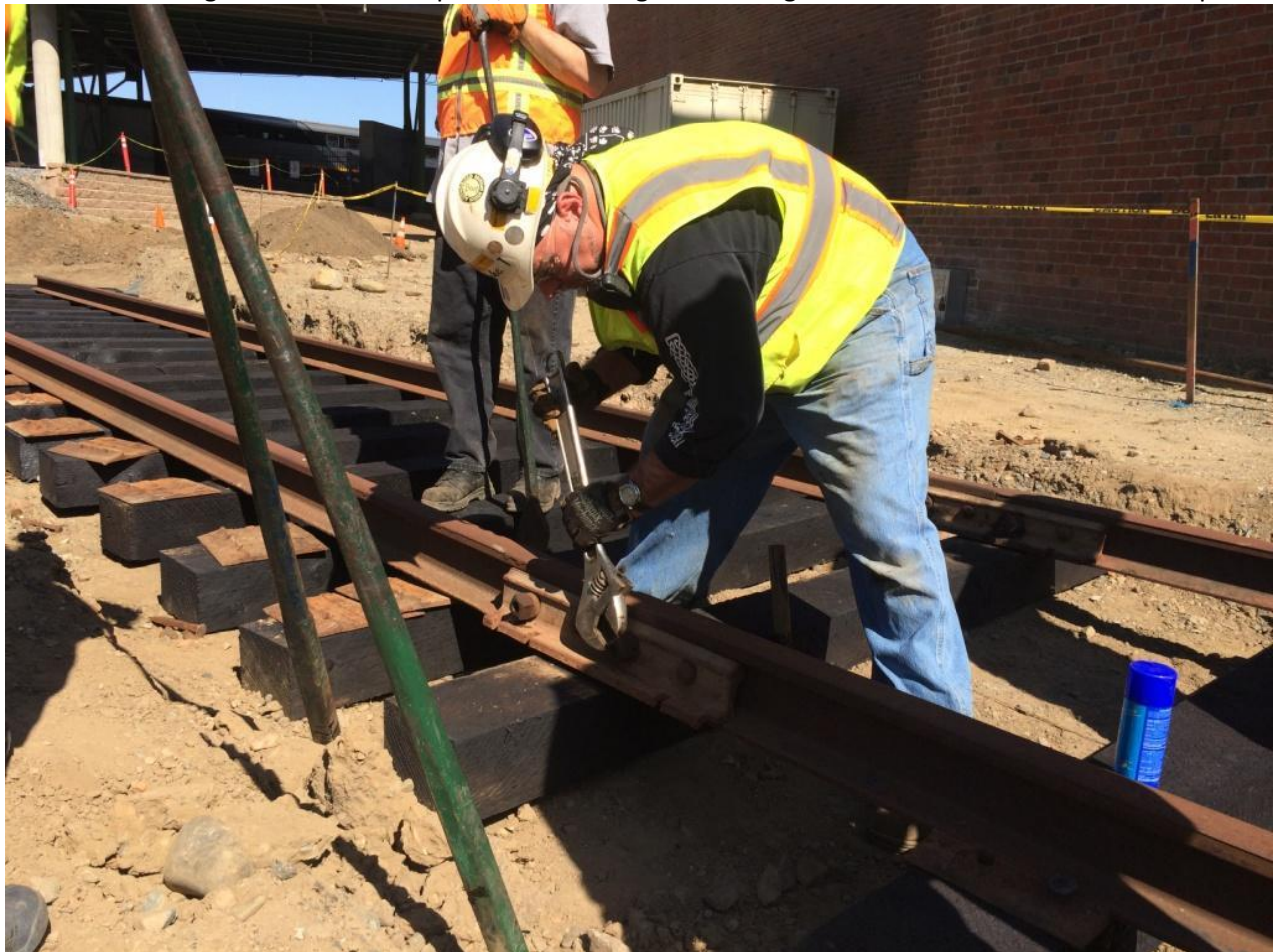
Mike F. bolts the rails together
