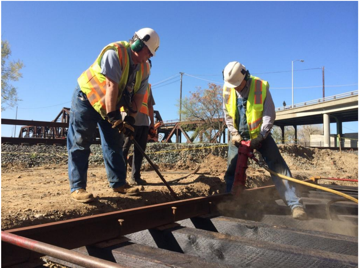
With both rails now in place, properly spaced, and plated, Chris nips the ties while Steve spikes
