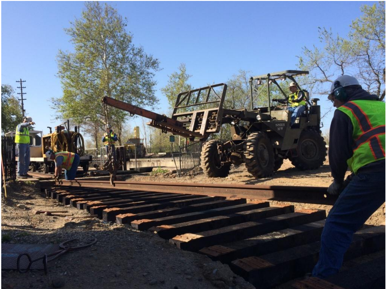
Chris and Steve place the first stick of rail with Mike F. on Big Green
