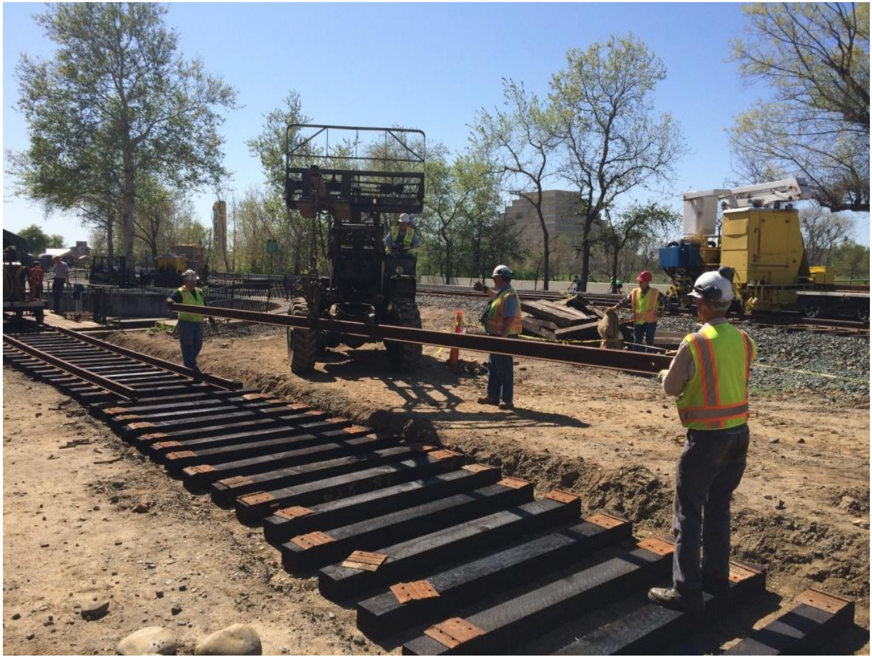
With the first segment of track complete, Steve in Big Green brings over the first rail for the second panel
