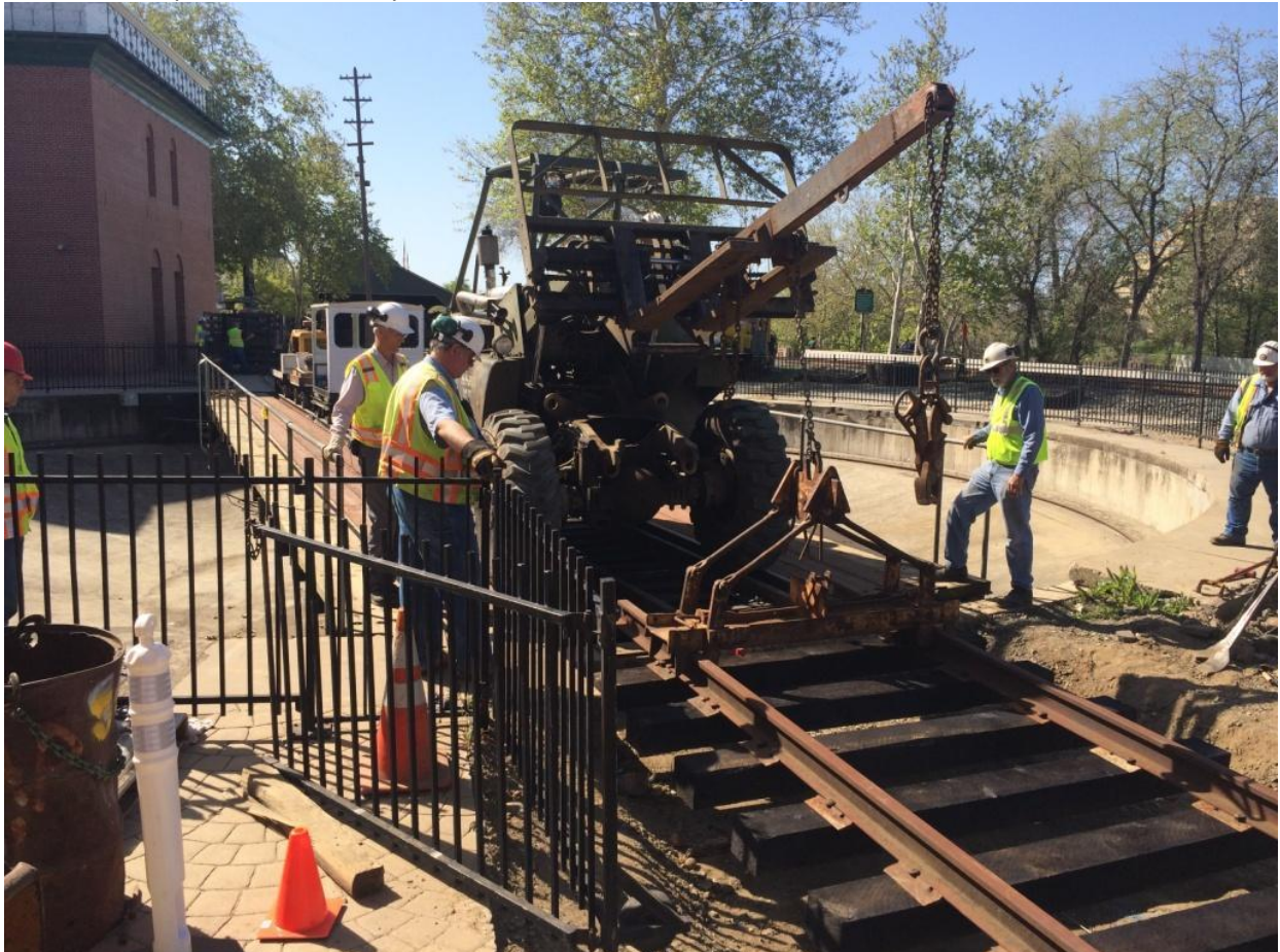
Now that the first panel is complete, we use the track lifter to lift the track up onto the concrete base of the turntable pit
