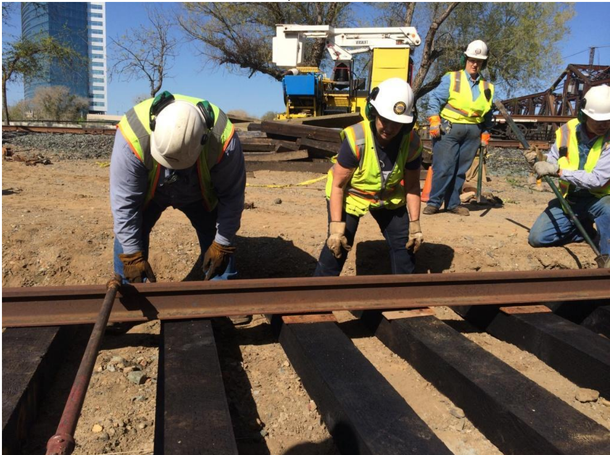
Frank and Pam gauge and plate the west rail
