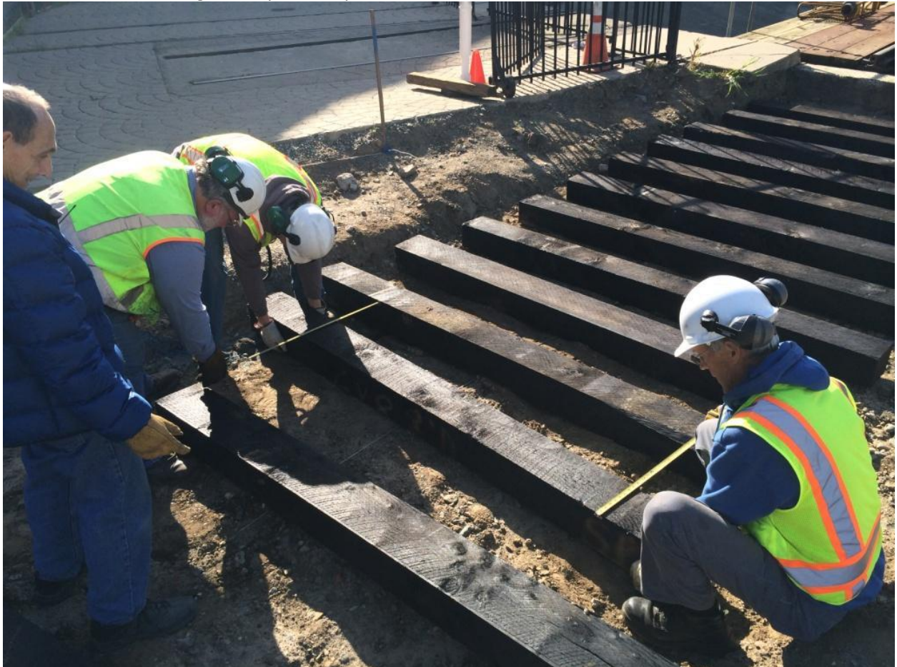
Harry G. guides the precision placement of ties by Frank, Steve, and Kent
